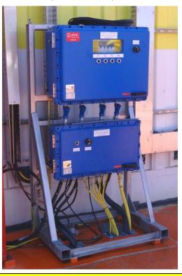
Control Panel suitable for floor installation, complete with mechanical support in AISI 316L stainless steel and prepared for the cable inlet from bottom, already installed on platform. Typical managing capacity:
