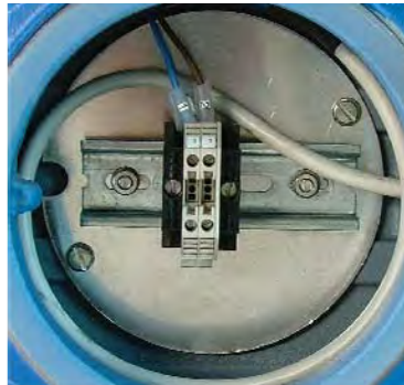
INTERNAL BASE PLATE LAYOUT OF GUB-02 + 1xFTC STANDARD TYPE (TYPICAL)
